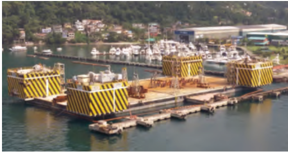
Figure 13 BrasFELS Floating Dry Dock
