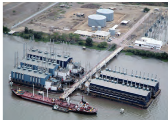
Figure 3 Power barges deployment in Ecuador
